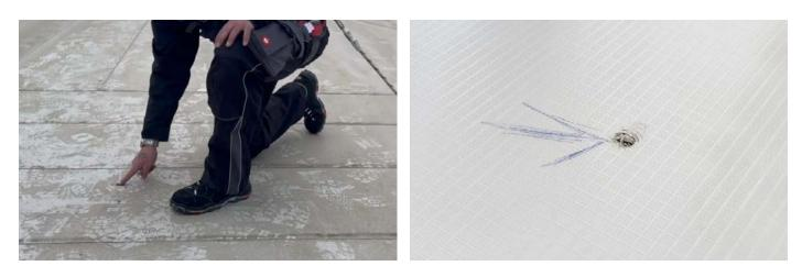
Repairs must be carried out using KÖSTER-approved systems and procedures. Any repair, regardless of scale, should be preceded by proper cleaning and preparation of the surface. Small punctures or cracks must be sealed using KÖSTER-compatible sealants or membranes, applied according to KÖSTER's technical data sheets and repair manual.
